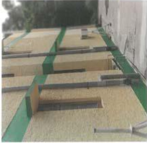
Pipe Lines Laying
