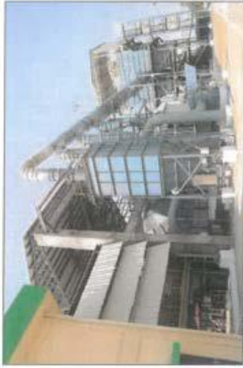
Installed Big Filters at Cement Silo
